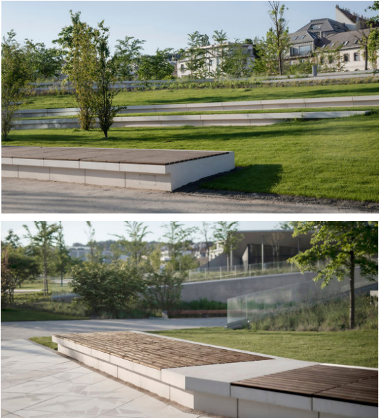
Timber top concrete retaining edge seating
