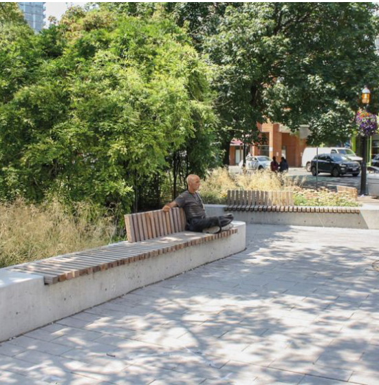
Timber top concrete retaining edge seating bench & back
