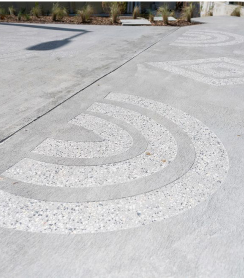
Sandblasting technique removes the top layer of concrete. This exposes the aggregate layer which displays the design
